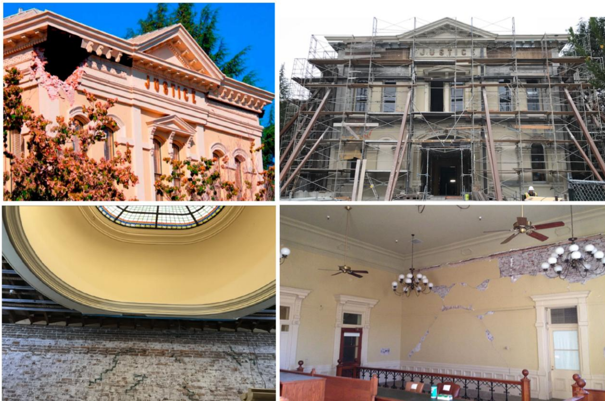
Fig. 4- Structural cracking of Napa County Historic Courthouse after 2014 South Napa Earthquake
